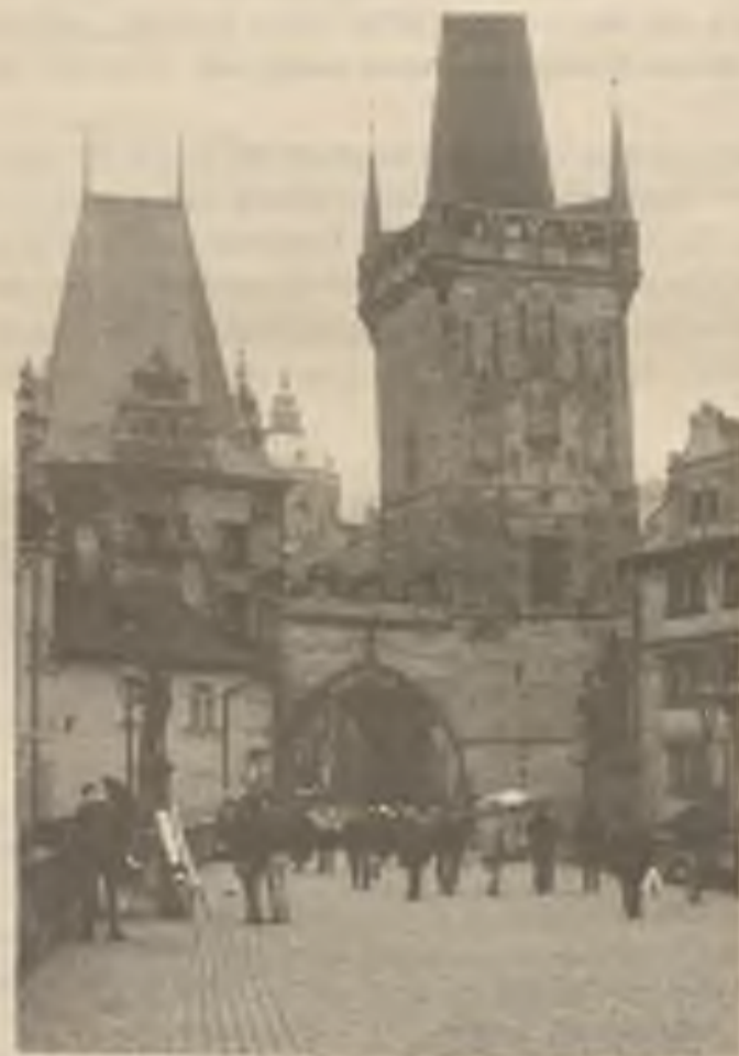
Charles Bridge in Prague .
