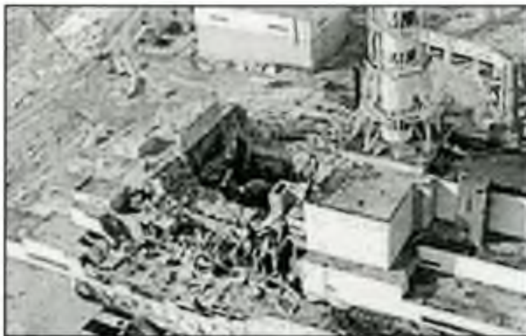
Nuclear reactor after the accident
