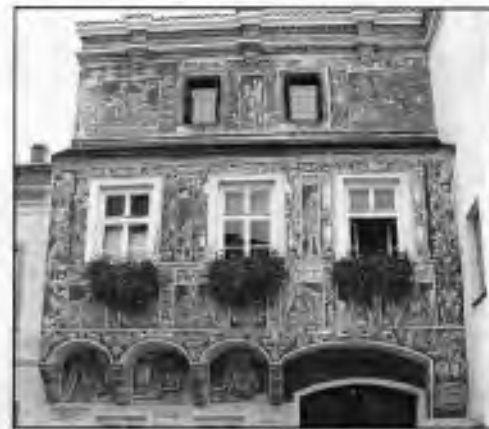
Sgraffito-decorated house in Slavonice
