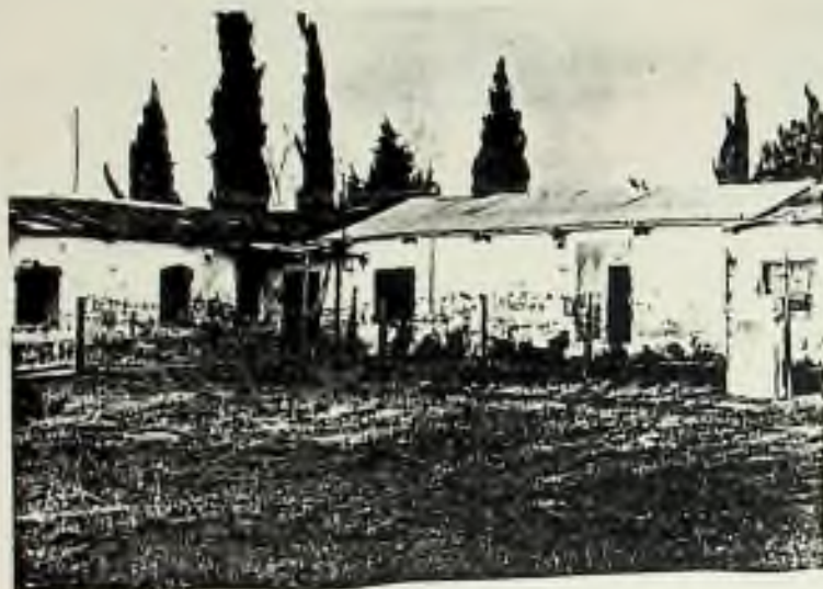
Camp Capua, near Naples: in these delapidated buildings on west side of the camp dozens of refugees live for several years, without hope. No windows, no doors ...
