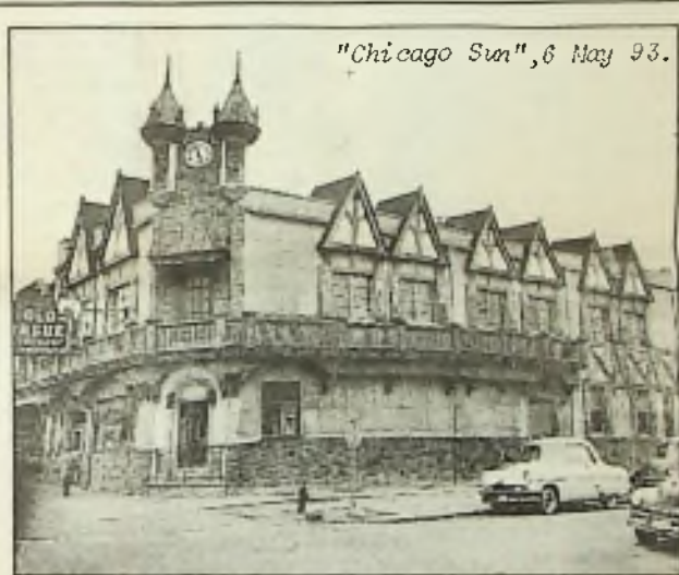
Fire caused extensive damage today to the Old Prague Restaurant in Cicero (shown in a 1956 photo).
