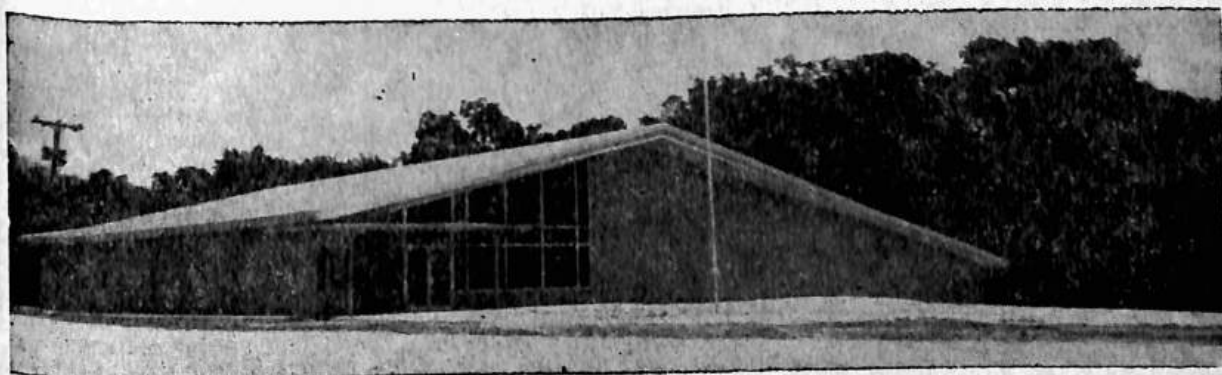
Sokol Žižka and S.P.J.S.T. Gymnasium and Recreation Center, Dallas, Texas.
