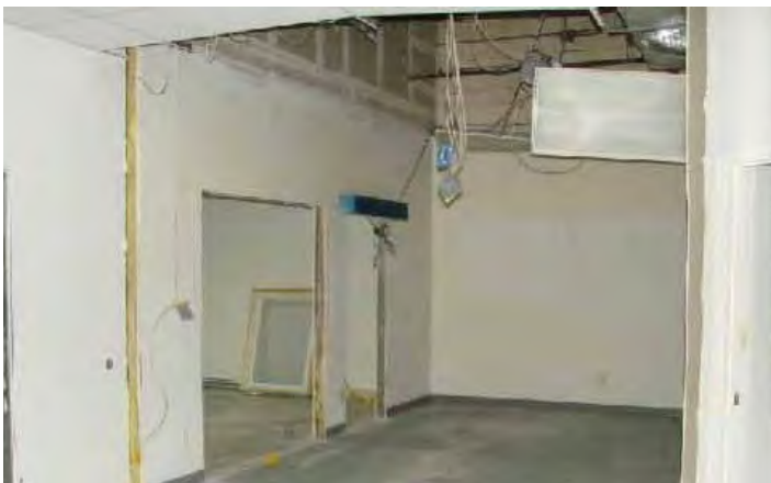
Demolition & Renovation of The New Hall
