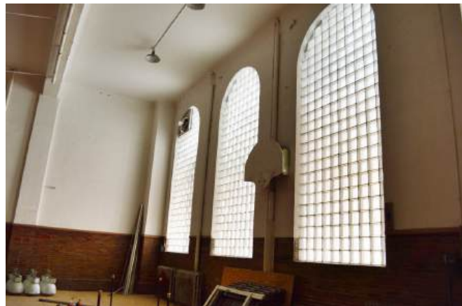
Immense windows line one side of the Sokol gymnasium, where developer Charles Jones envisions a ground-floor restaurant. (photo/Cindy Hadish)
