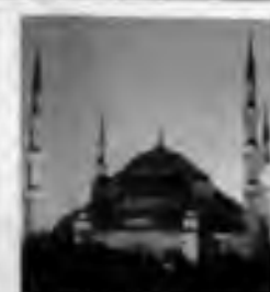
Construction of Istanbul's Blue Mosque
